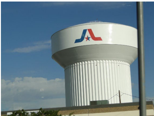
Water tank (Arlington, TX) (allikas: Ref #12).
