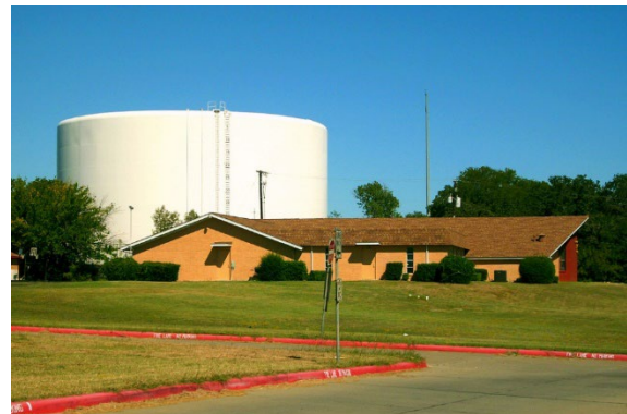
Water tank (North Richland Hills, TX) (allikas: Ref #13).
