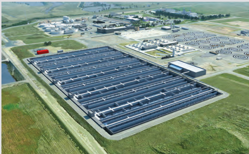
The Biological Nutrient Removal Facility at EchoWater is using BIM in pioneering ways across the project lifecycle.
