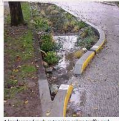
A landscaped curb extension calms traffic and captures and infiltrates street runoff in Portland, Oregon.
